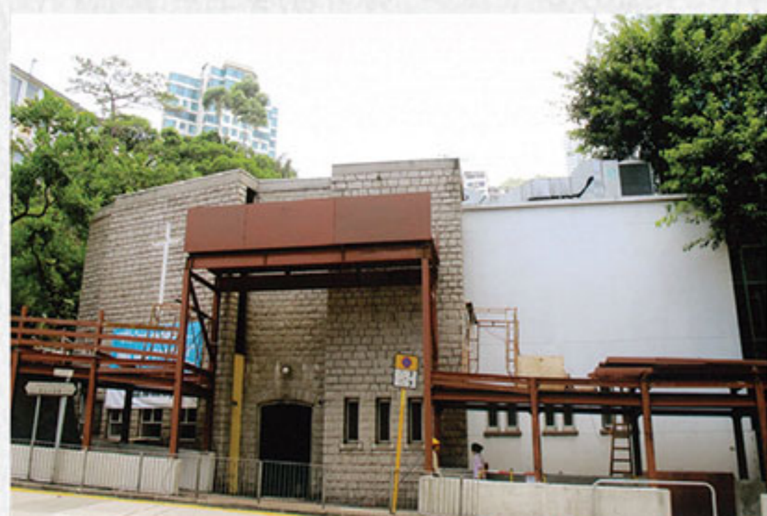
Hoarding works - Sep 2014
