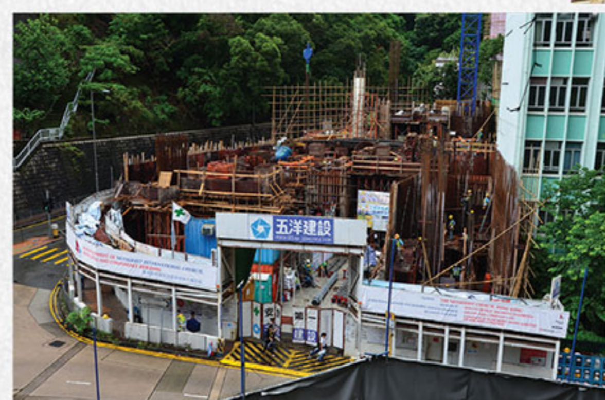
Construction of G/F - Jul 2016
